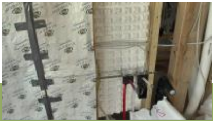
PCM mats had to be resized in walls to 24"x16" to fit the framing.
