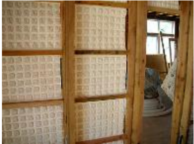
PCM mats had to be resized in walls to 24"x16" to fit the framing.
